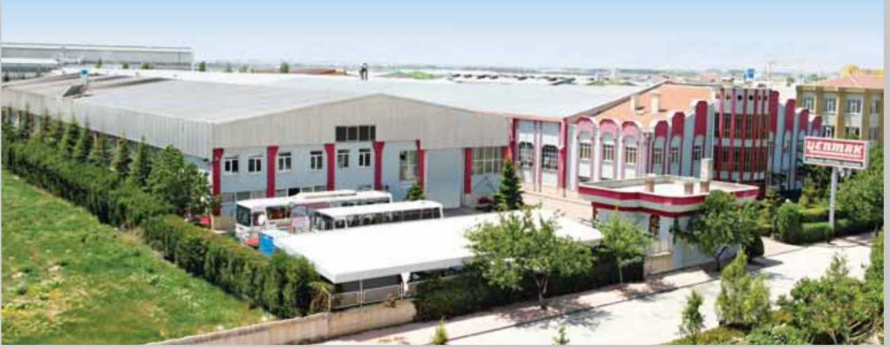
PISTON & PISTON PIN PRODUCTION FACILITY / PİSTON VE PİSTON PİMİ ÜRETİM TESİSİ
